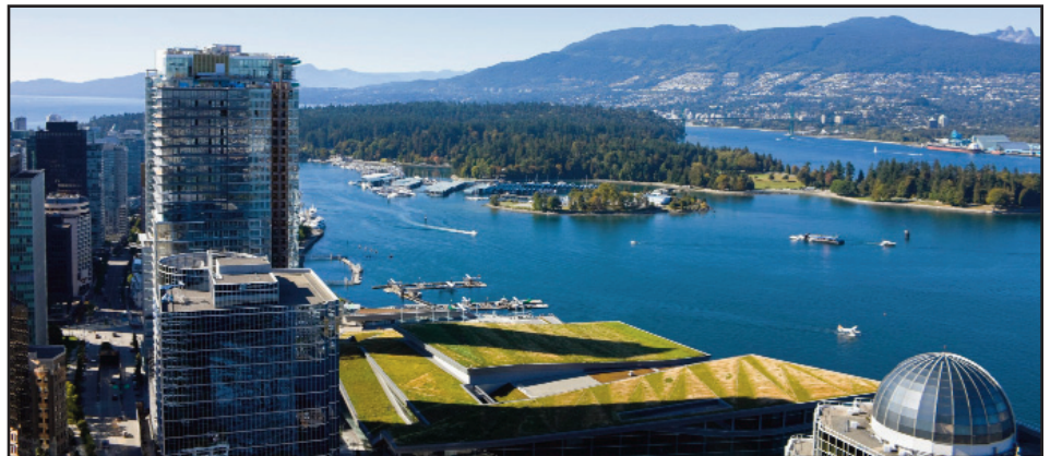
The Vancouver Convention center and its green roof.
